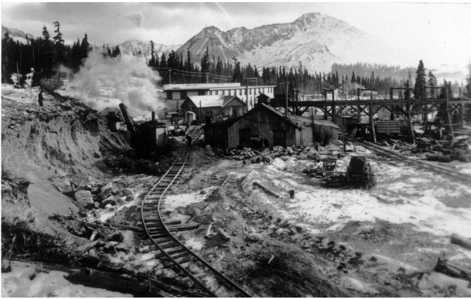
Figure 69. Mine and mill , photograph, 1940, Denver Public Library Digital Collections (X-60993), https://digital.denverlibrary.org/digital/collection/p15330coll22/id/36912/rec/1 .
